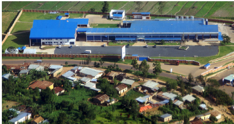
Fig. 1.2 Inyange factory at Masaka, Kigali
