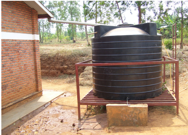
Fig 9.6: A water tank
