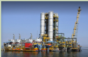
Picture 2.1: Kivu watt power station
