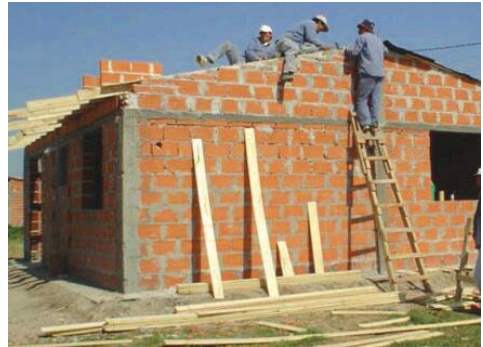
A house that is being built with bricks, cement and sand
