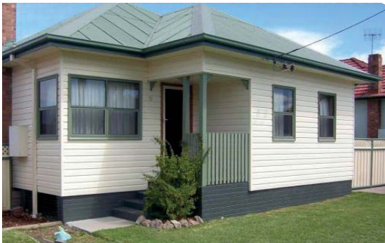
A house built with boards and iron sheets
