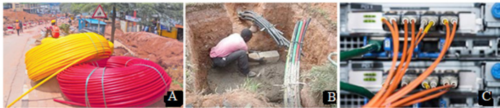
Fig.5. 1: The installation and use of optical fiber in Rwanda
