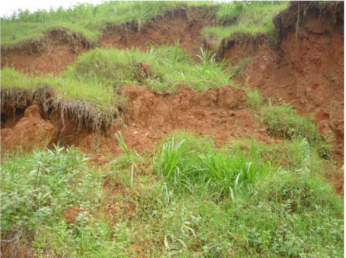
Figure 7. 128 Landslide in Gakenke district
