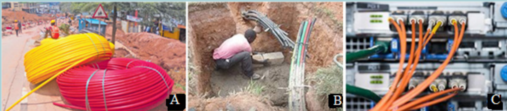
Fig.3. 1: The installation and use of optical fiber in Rwanda
