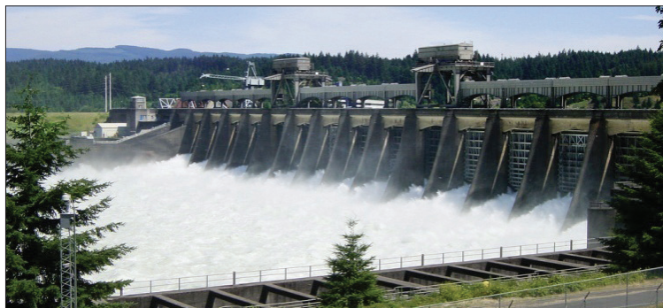
Figure 6.14: Hydroelectric power station
