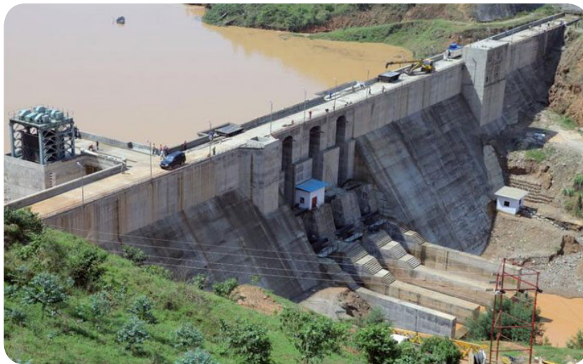
Hydroelectricity power dam along River Nyabarongo, Rwanda
