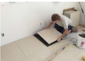
Tiled mud floor (floor covered by tiles.)
