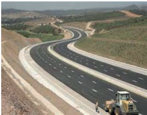
Construction of new roads
