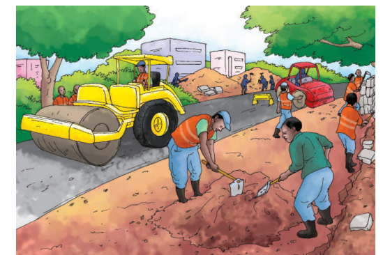
Construction of roads
