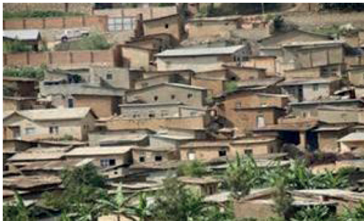
Slum area (Bad housing)
