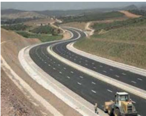
Construction of new roads
