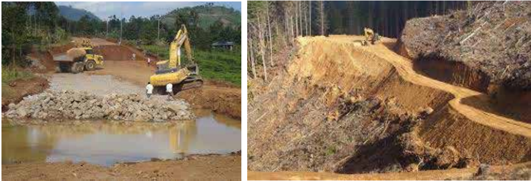
Figure 3.78. Construction of roads in swampy and sloppy areas
