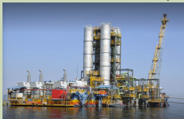
Picture 2.1: Kivu watt power station
