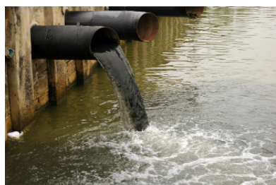
Fig. 12.9: Water contaminated with sewage waste
