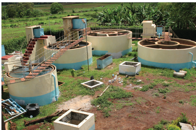
Fig 7.4 Water treatment plant in Rwanda
