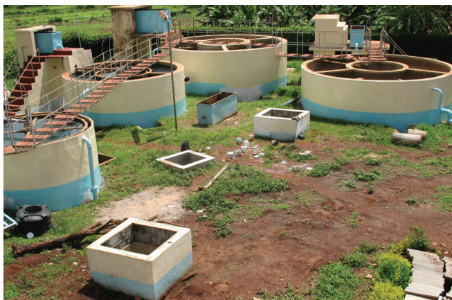
Fig. 1.5 A Water Treatment Plant in Rwanda
