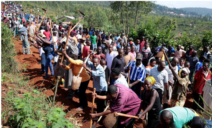
Figure 5: Rwandans unite in 'Umuganda' (community work)
