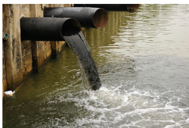
Fig. 12.9: Water contaminated with sewage waste
