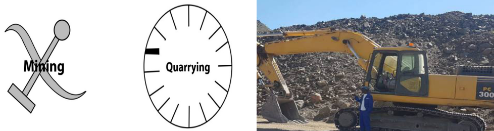
Mining area, quarrying and machine in mining activities
