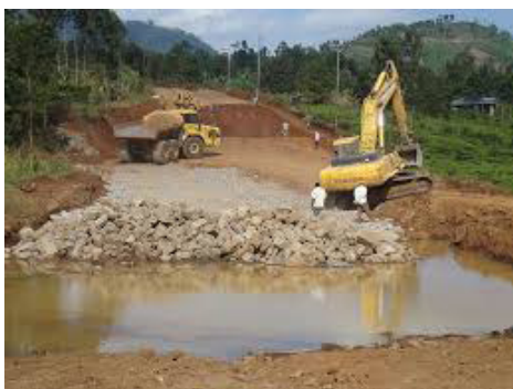
Construction of roads in swampy and sloppy areas
