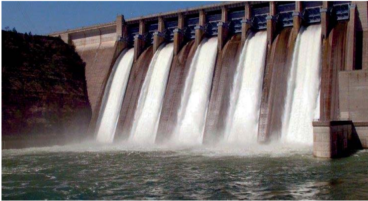
Fig 14.5 Rusizi hydropower station
