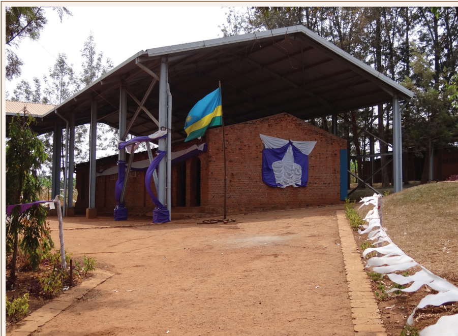
Figure 1: Ntarama Genocide Memorial site in Bugesera, Rwanda
