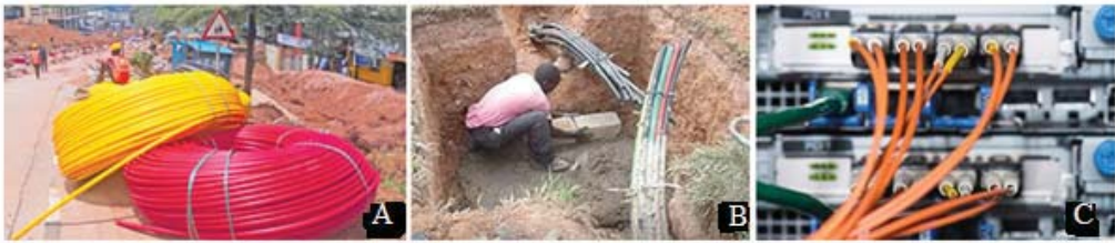
Fig.6. 1: The installation and use of optical fiber in Rwanda
