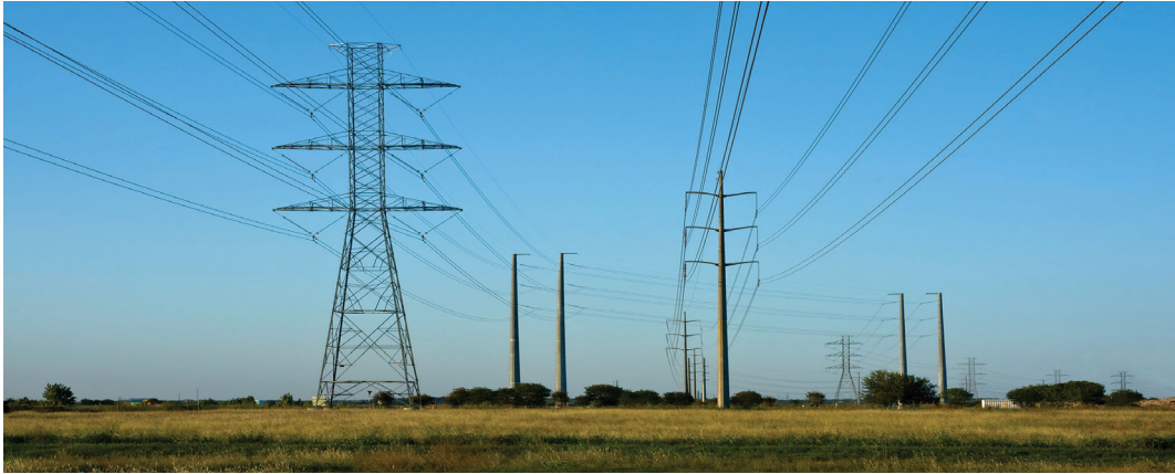
Fig. 8.15: Pylons and electricity transmission cables
