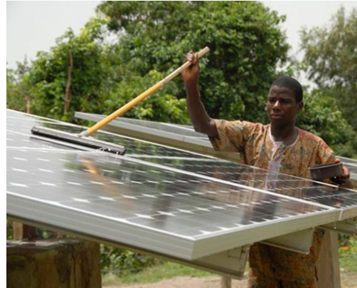
(b) Cleaning solar panel
