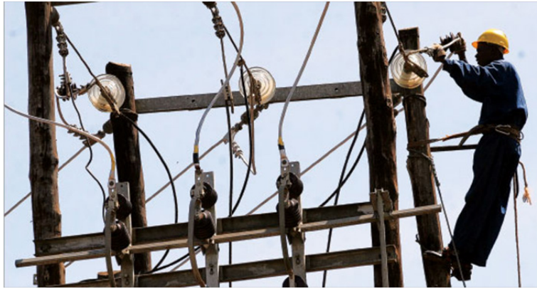
Fig. 4.6: Higher capacity transmission lines being set up
