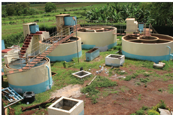
Fig 7.4 Water treatment plant in Rwanda
