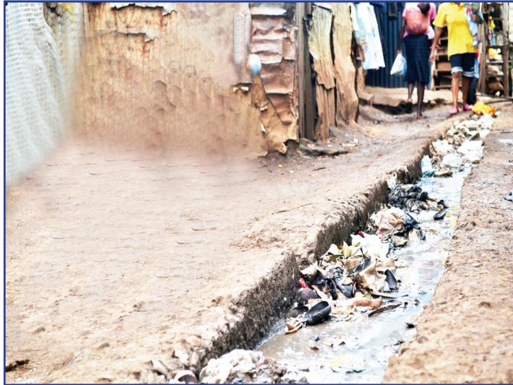
Figure 4.12: Open sewage and sanitation conditions.
