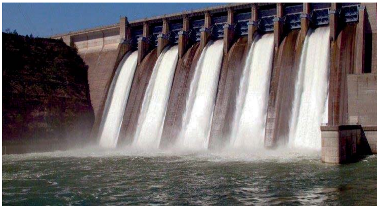
Fig 14.5 Rusizi hydropower station
