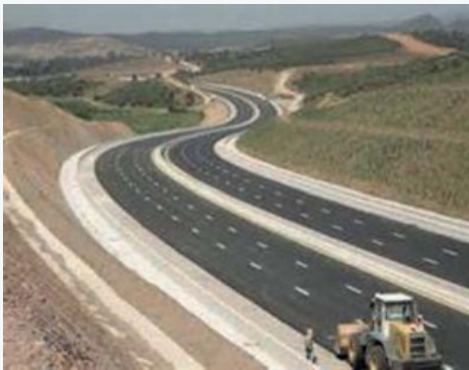
Construction of new roads
