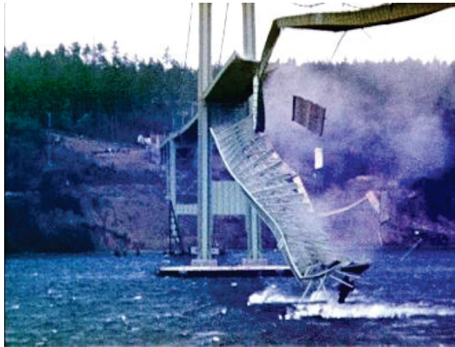
Fig.3-16; Vibrations breaking the bridge
